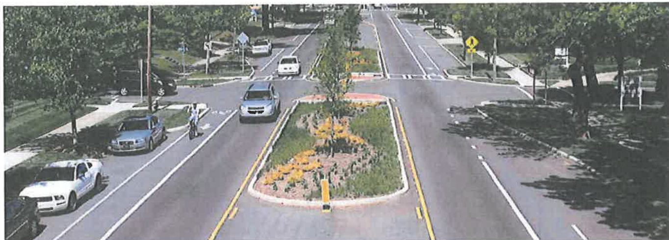
In addition to making East Boulevard in Charlotte, N.C., more attractive, a road diet reduced travel speeds, bicycle and pedestrian injury rates and the number of rear-end and left-turn collisions. Photo courtesy city of Charlotte
