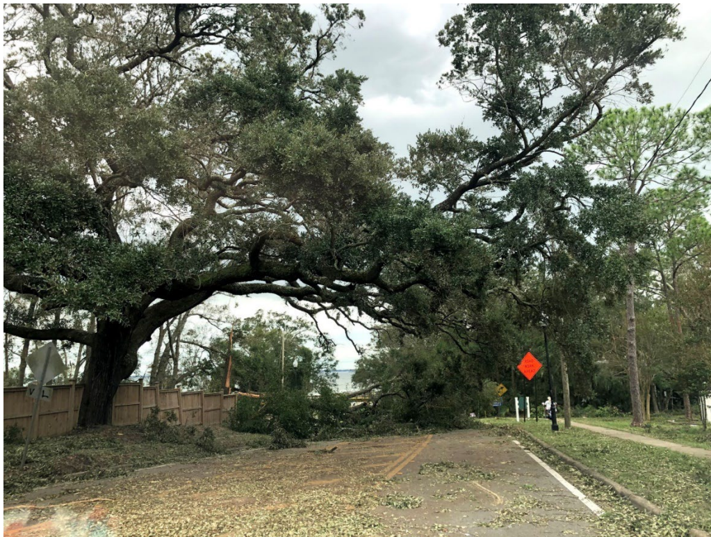
Figure 5: Tree damage in Pensacola from Hurricane Sally 19
