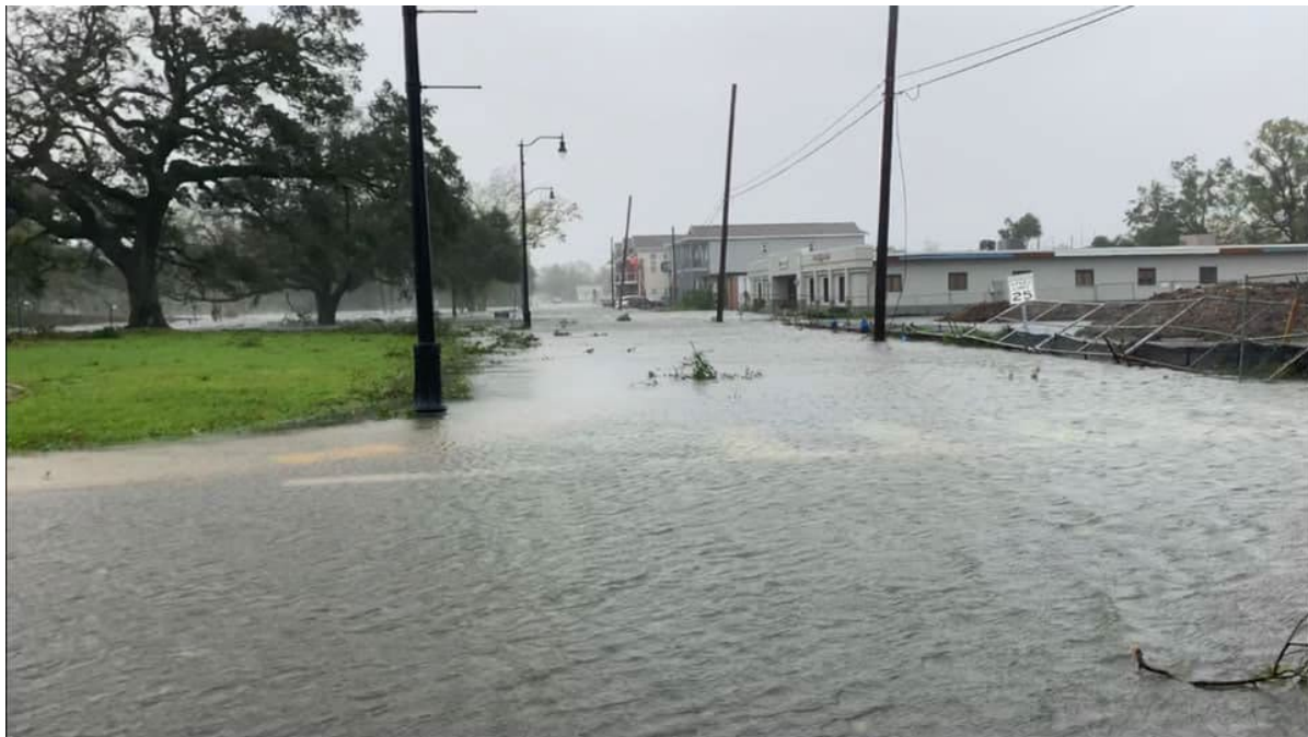
Figure 10: Inland flash flooding in Pensacola during Sally 30
