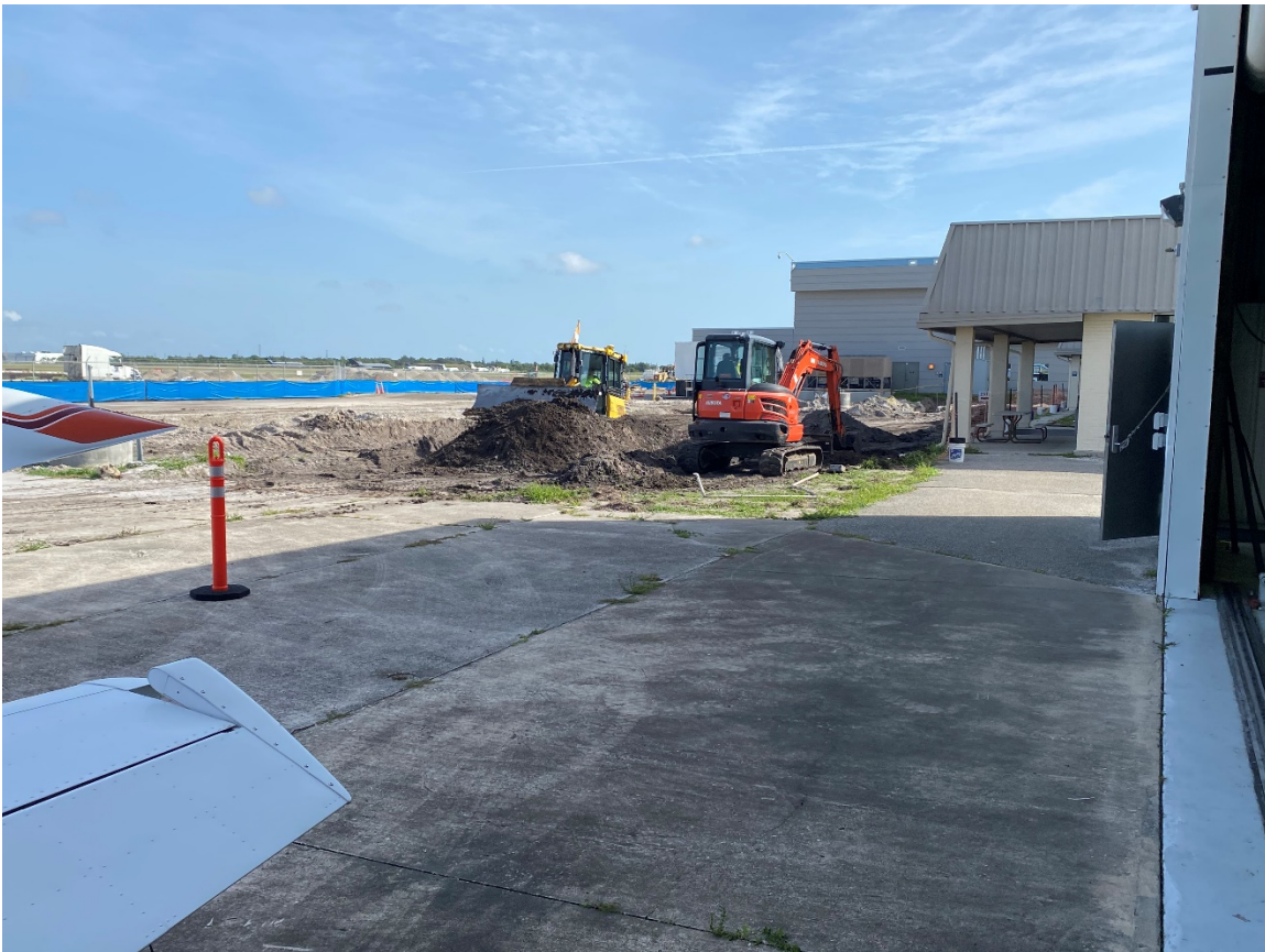
Picture 1 Airport construction outside of EFSC Aviation Center
