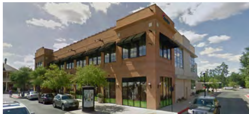
Example of simple, but well-executed building massing expressing floors, columns, foundation, and wall plane variation
