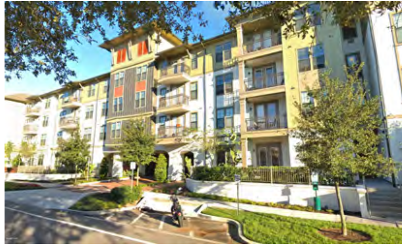
Example multi-family facade creating interest through variations in solid and void composition, color, material, and height.
