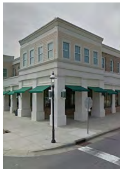
Example of proper building proportioning and clear delineation between ground floor and upper levels.
