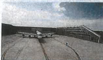
Milwaukee (USA) Project Highlight: Facility was installed directly on existing aircraft pavement.
