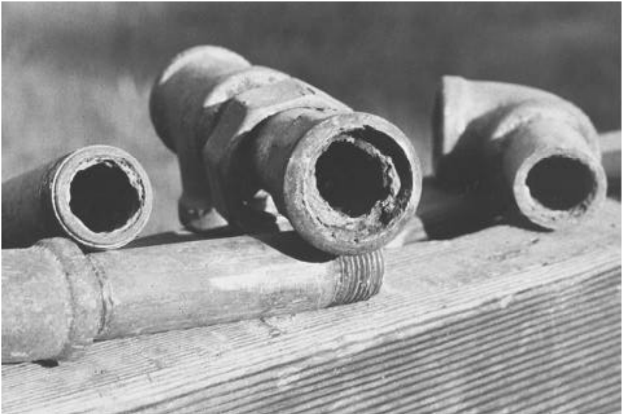
Galvanized pipe sections removed from an older house. Mineral deposits and corrosion within the pipe had severely reduced water flow to the plumbing fixtures.
