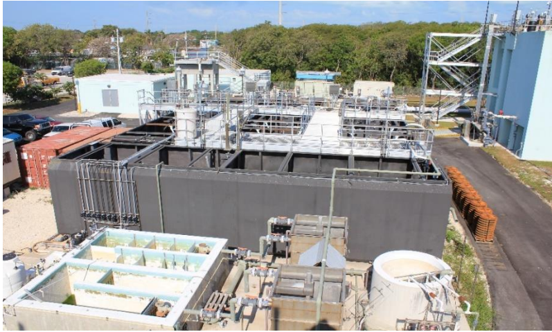
Key Largo Wastewater Treatment District Facility (Source: Barbara Powell)
