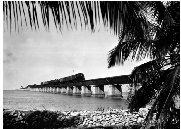
Florida East Coast Railway train traveling overseas bridge Knight Key, Florida
