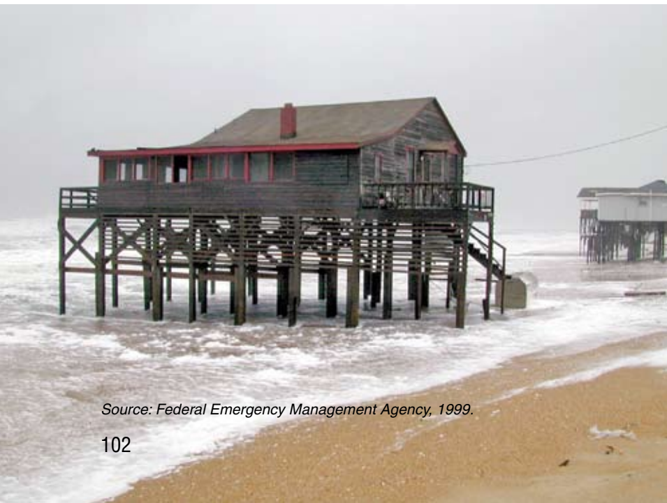
Figure 5.11: Elevation on piles in the V-zone.
