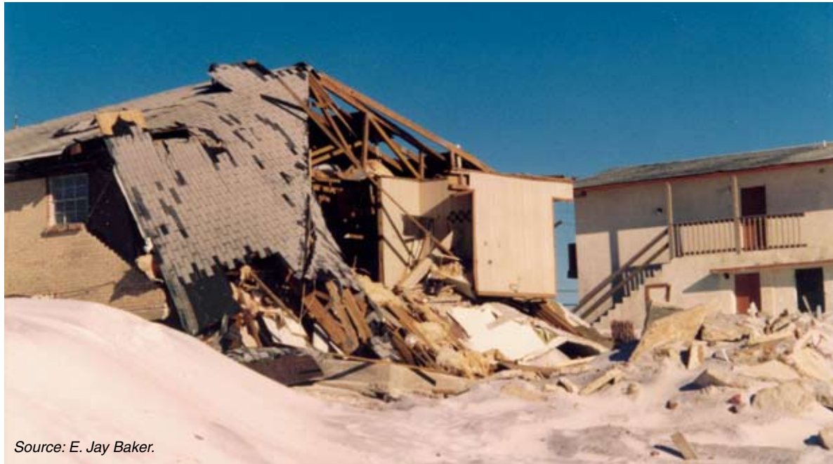
Figure 5.4: Storm surge damage from Hurricane Opal.
