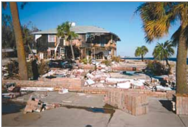
Photo (above left): Homes along Pensacola Bay show the fury of Hurricane Ivan's winds and storm surge. Waves reaching 20 to 30 feet leveled the home in the foreground, leaving only the foundation. The home in the background also sustained catastrophic damage. FEMA Photo/Butch Kinerney (September 20, 2004, Pensacola, Florida).
