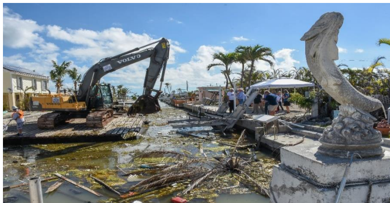
Canal cleanup following Hurricane Irma (Source: B. Powell)
