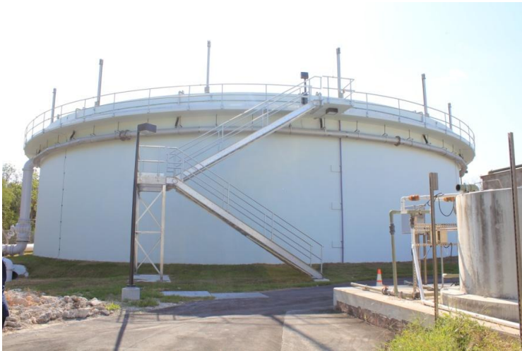
Key Largo Wastewater Treatment Plant
